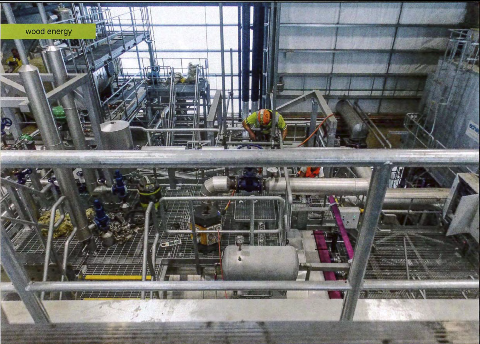
The inner workings of the Burwood Hospital chip boiler set-up.
