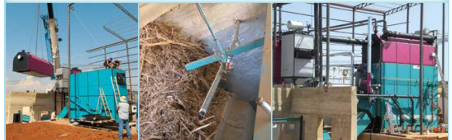
Hot water boiler • Combustion system: Water-cooled reciprocating grate • Fuel: Wood chips, bark and roots Commissioned in 2010
