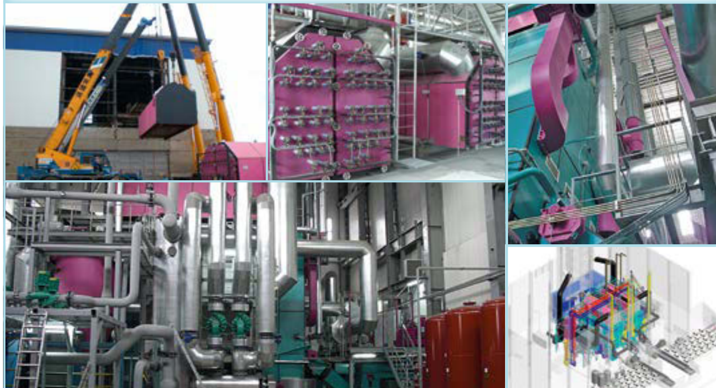
2 x 10,000 kW - Superheated water boiler plant, 115°C, process heat • Combustion system: Water-cooled reciprocating grate Fuel: Wood chips and bark • Commissioned in 2009
