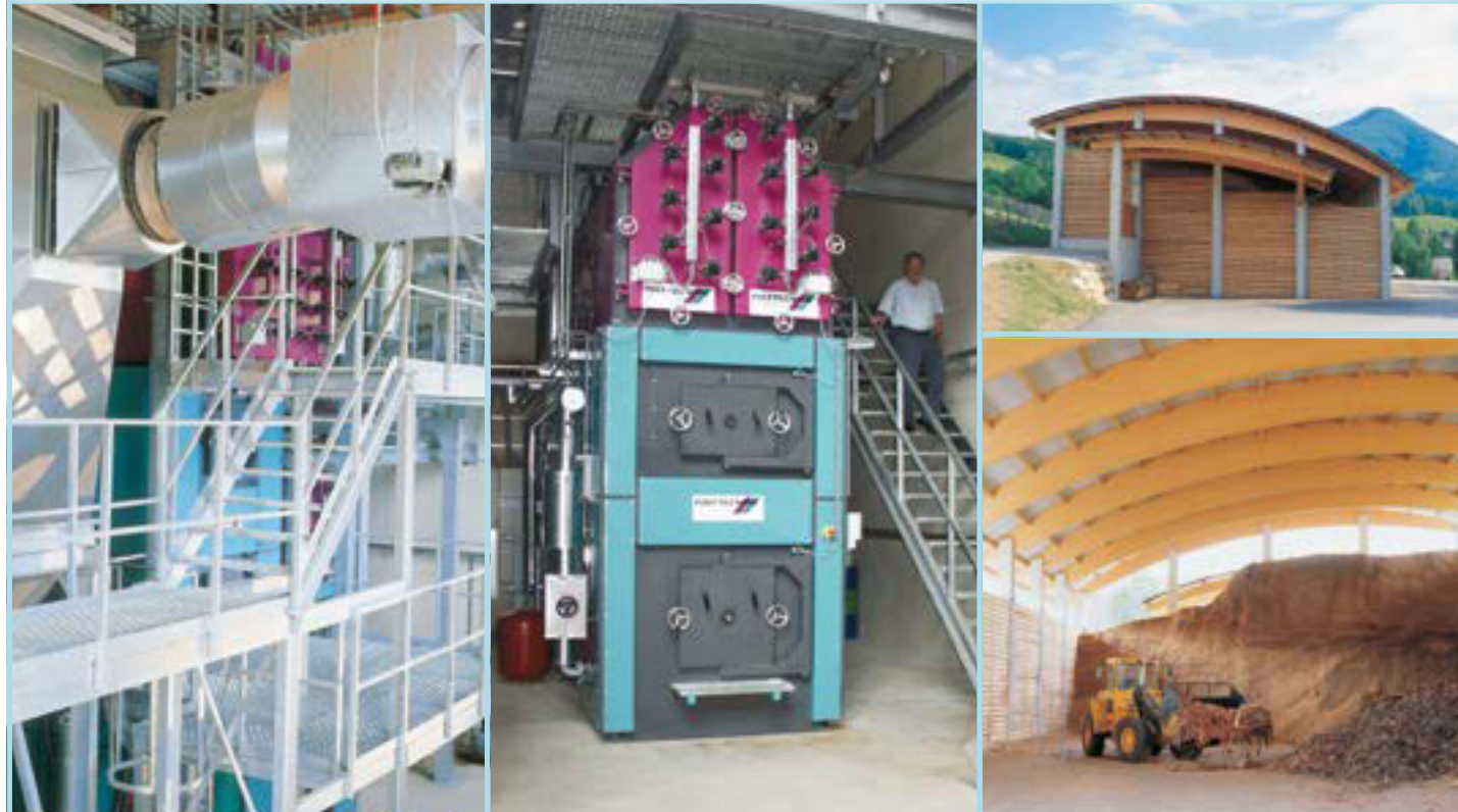
Combustion system: Water-cooled reciprocating grate • Fuel: Wood chips, forest residues and bark • Commissioned in 2002
