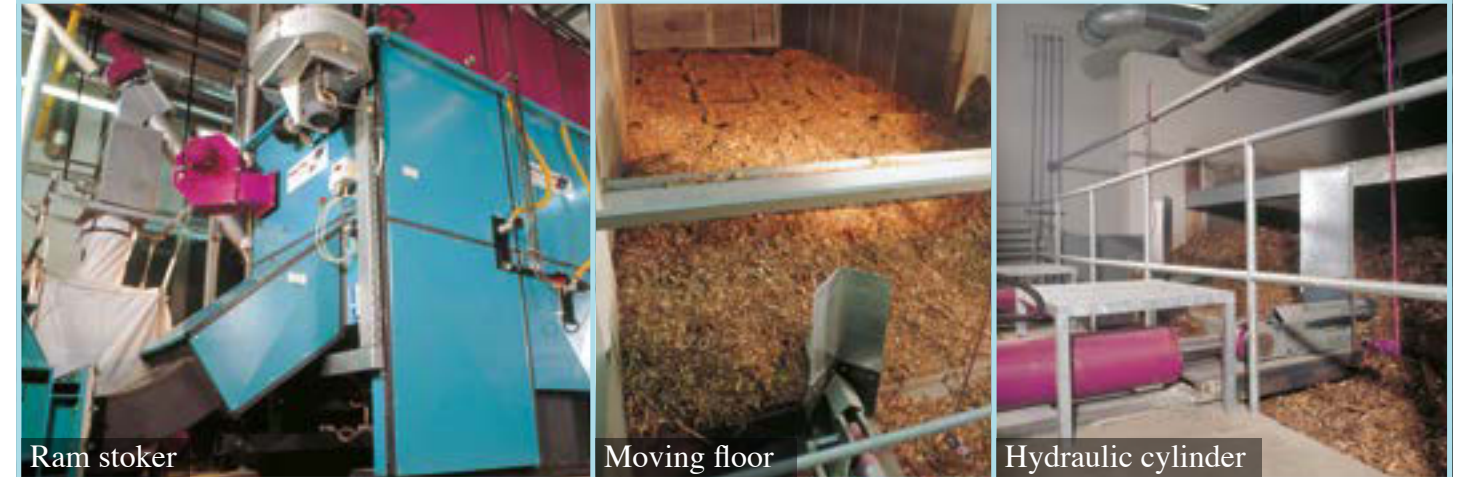
Combustion system: Water-cooled reciprocating grate • Fuel: Wood chips and forest residues • Commissioned in 2001
