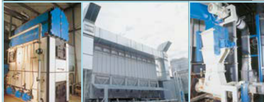
Combustion system: Underfeed stoker • Fuel: Wood processing residues like fines, saw dust and wood chips Commissioned in 2000
