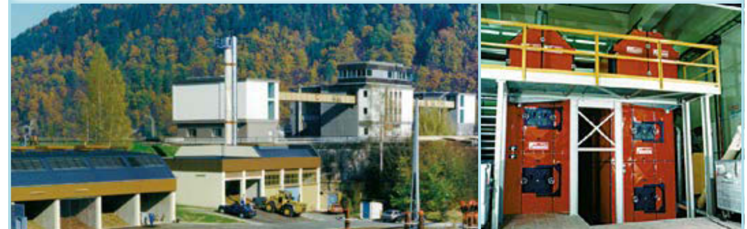
Combustion system: Water-cooled reciprocating grate • Fuel: Drift wood, bark and wood shavings Commissioned in 1990
