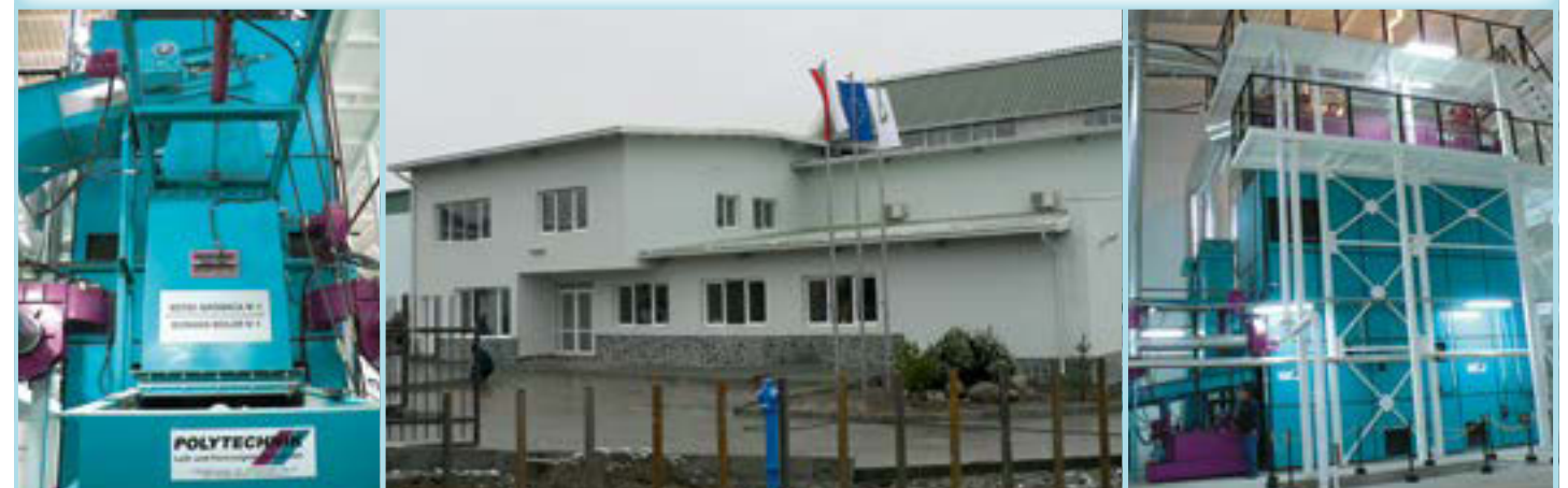
2 x 5,000 kW - Superheated water boiler plant, 110°C • Combustion system: Water-cooled reciprocating grate Fuel: Wood chips and bark • Commissioned in 2007
