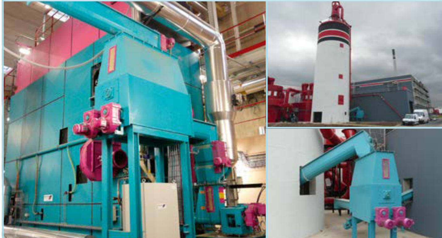
Combustion system: Underfeed stoker with water-cooled reciprocating grate • Fuel: Wood chips from particle board Commissioned in 2008
