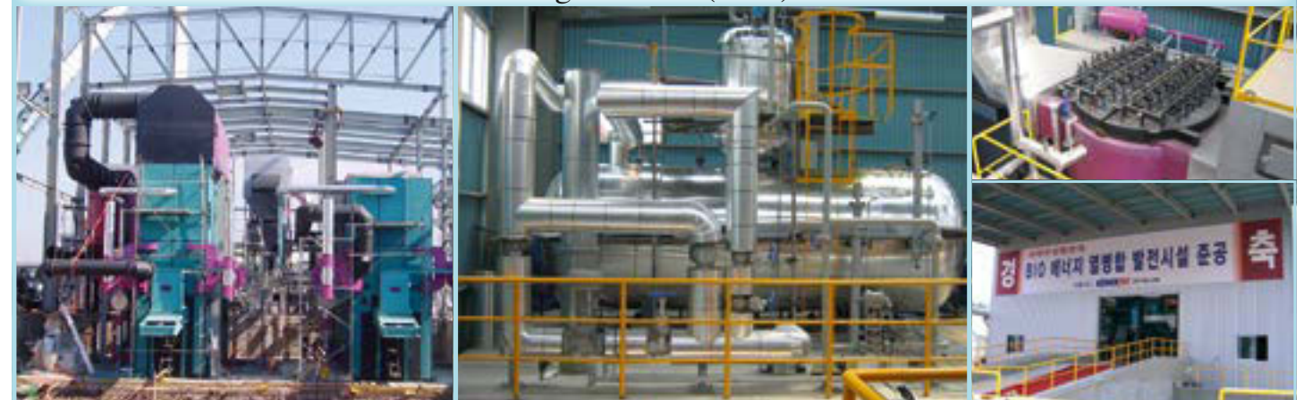
2 x 8,700 kW - Superheated steam boiler plant, 28 bar / 430°C with two 750 kW steam turbine generators and 3 x 7,000 kW saturated steam boilers, 8 bar / 180°C • Combustion system: Water-cooled reciprocating grate • Fuel: Wood chips • Commissioned in 2005
