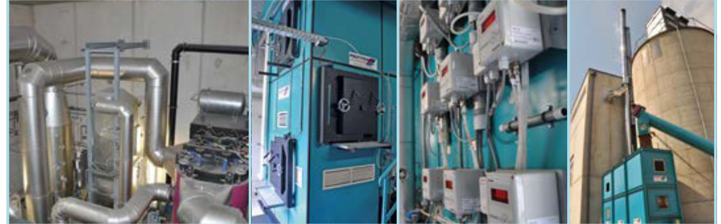
Boiler plant with dual fuel feeding system to run trials on different fuels Emission control system with additive dosing, scrubber and bag house
