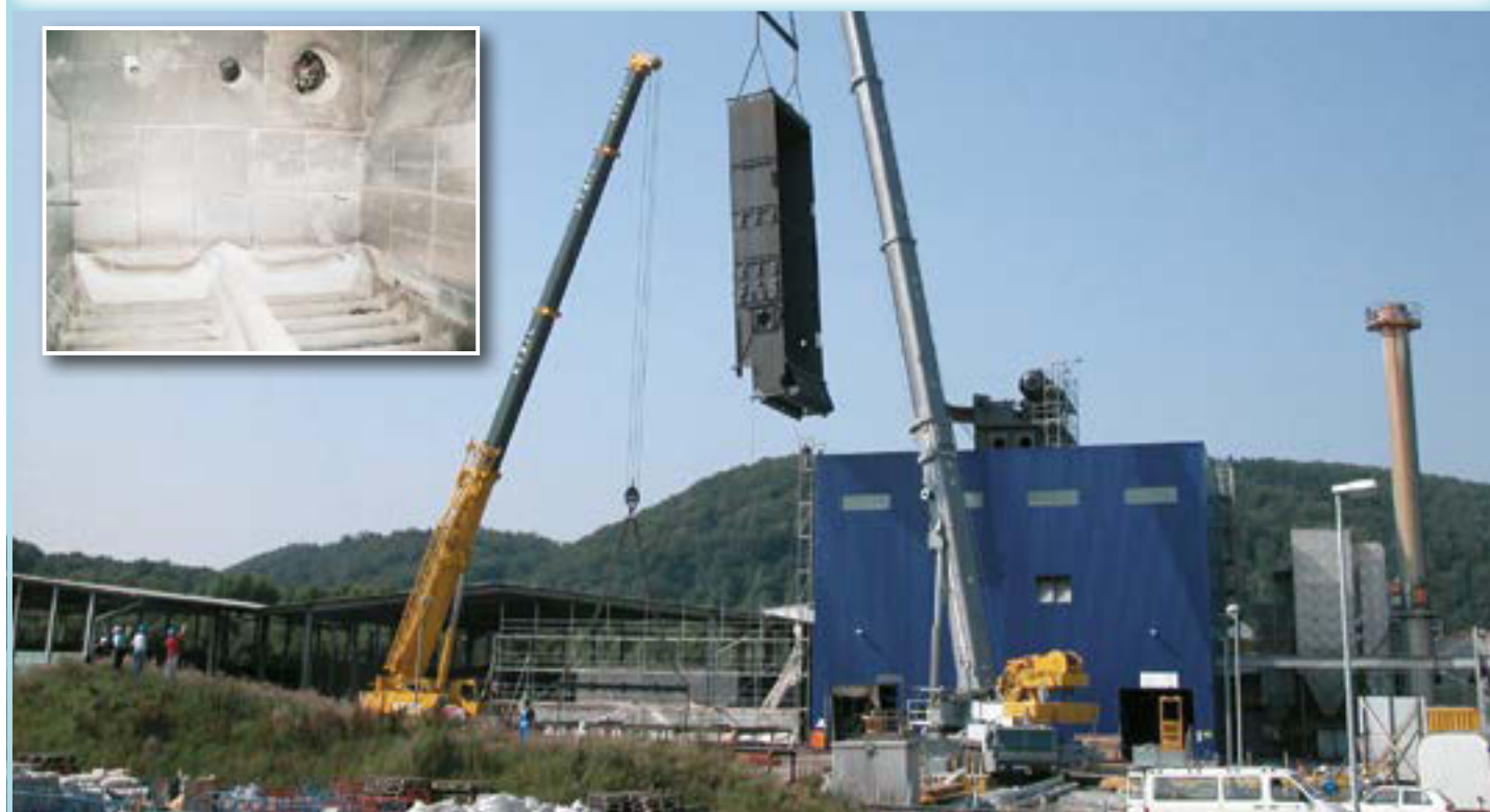
Superheated steam boiler, 63bar / 450°C • Combustion system: BFB bubbling fluidised bed boiler • Fuel: Construction and demolition wood, recycling residues • Emissions guarantees in accordance with 17. BImSchV • Commissioned in 2003
