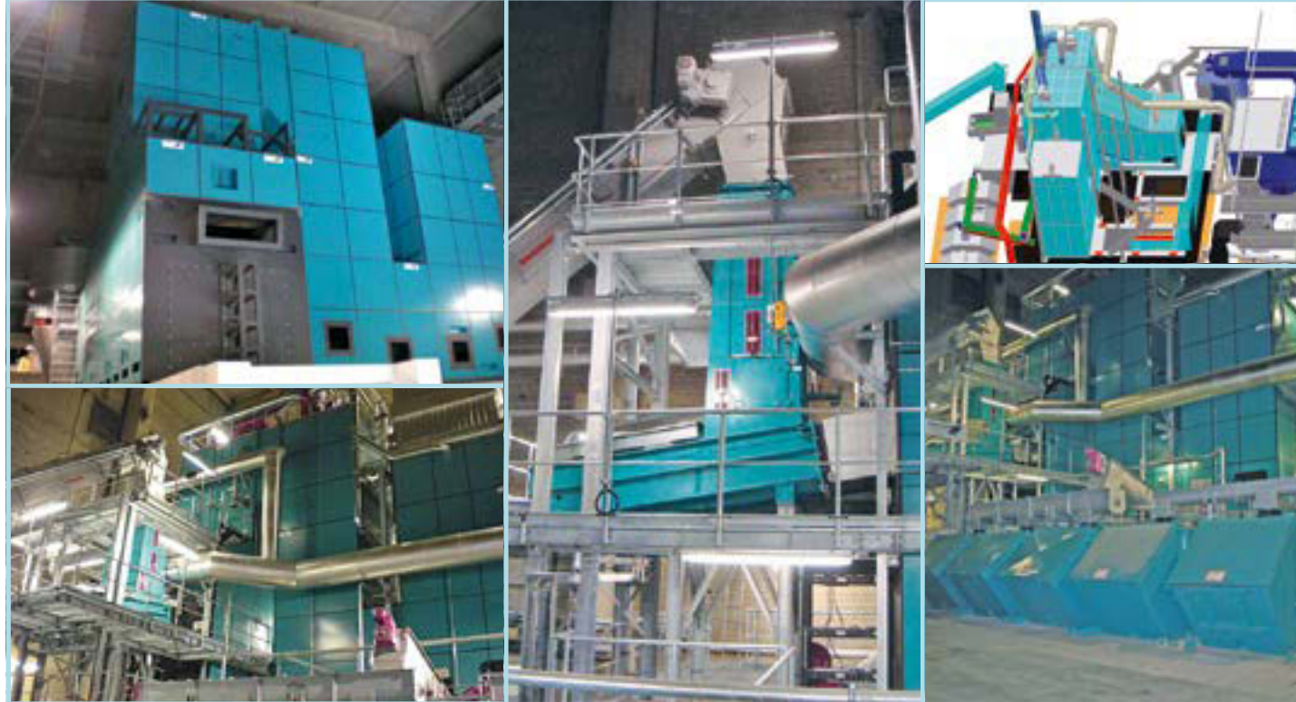
Superheated steam boiler, 60 bar / 430°C, steam extraction for district heating • Combustion system: Water-cooled reciprocating grate • Fuel: Compost rejects, wood chips and bark • Commissioned in 2011
