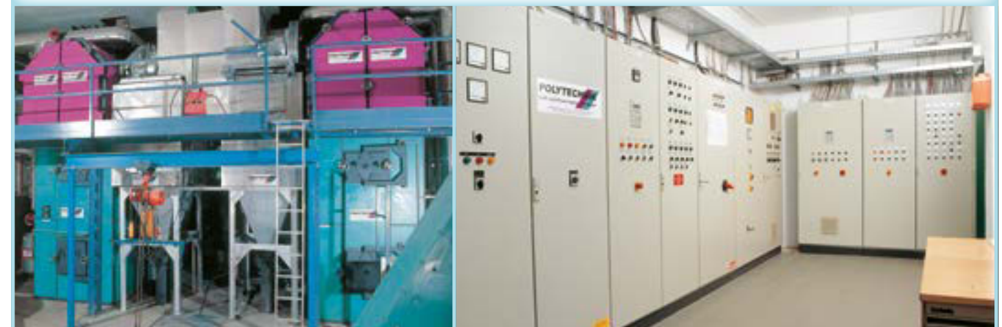
Combustion system: Water-cooled reciprocating grate • Fuel: Bark, wood chips and forest residues • Commissioned in 1994
