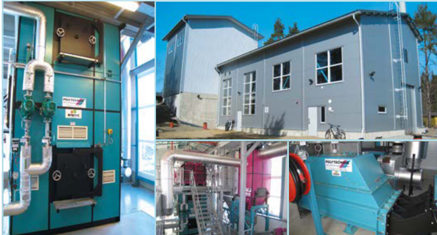
Superheated water boiler, 10 bar / 120°C • Combustion system: Water-cooled reciprocating grate Fuel: Wood chips, bark and peat • Commissioned in 2011
