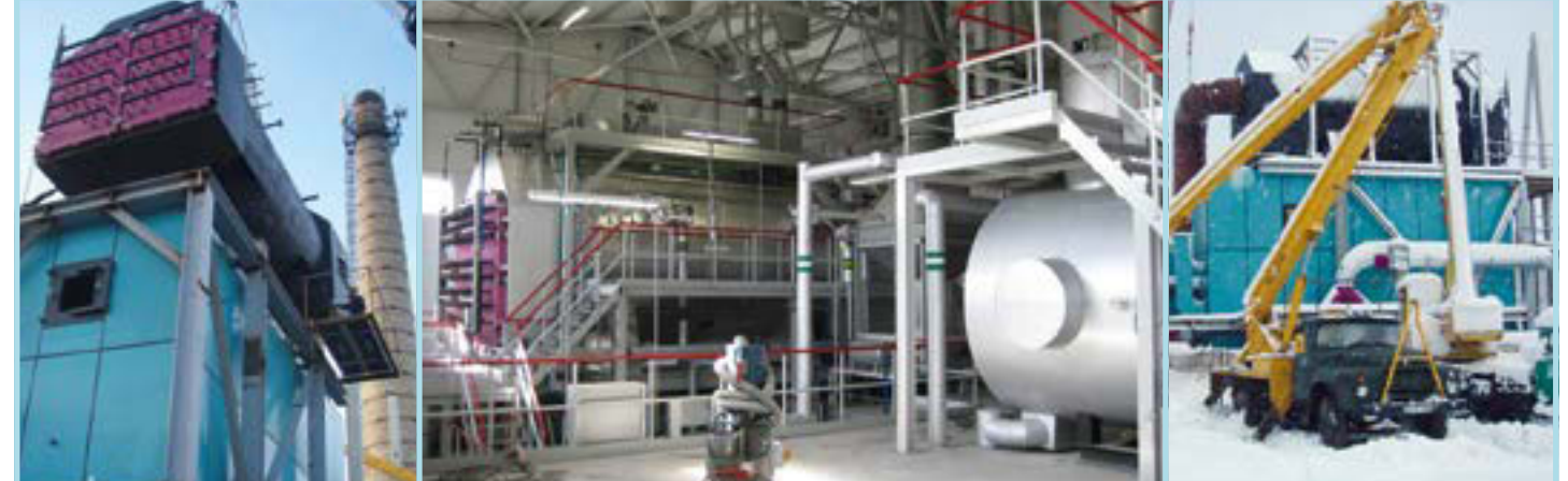
Saturated steam boiler, 12 bar / 190°C / 18t/h • Combustion system: Water-cooled reciprocating grate Fuel: Wood chips and bark • Commissioned in 2009
