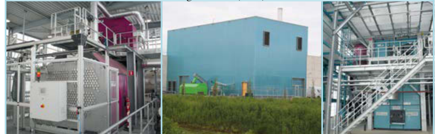
11.5 t/h superheated steam boiler, 29 bar / 250°C • Combustion system: Water-cooled reciprocating grate Fuel: Bark and construction and demolition wood • Commissioned in 2005
