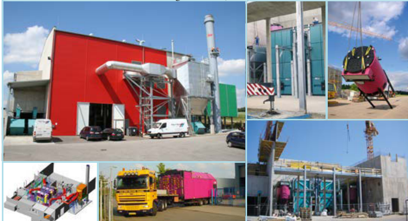
2 x 10,700 kW - Superheated steam boiler plant, 23 bar / 420°C • Combustion system: Water-cooled reciprocating grate Fuel: Wood chips, bark and saw dust • Commissioned in 2007
