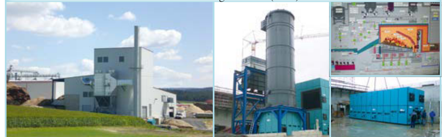
Thermal oil boiler plant with ORC turbine generator • Combustion system: Water-cooled reciprocating grate Fuel: Wood chips, bark, saw dust and roots • Commissioned in 2007
