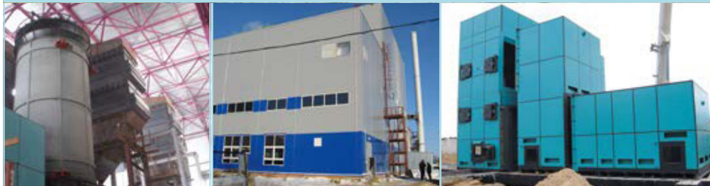
2 x 12,000 kW - Thermal oil boiler plant with 2 x 2,114 kW ORC turbine generators incl. district heating Combustion system: Water-cooled reciprocating grate • Fuel: Peat briquettes, wood chips and bark • Commissioned in 2011
