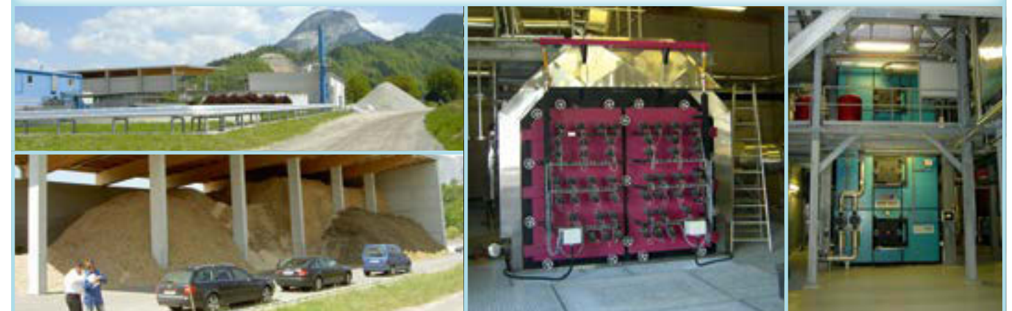
Combustion system: Water-cooled reciprocating grate • Fuel: Wood chips, bark and saw dust • Commissioned in 2007
