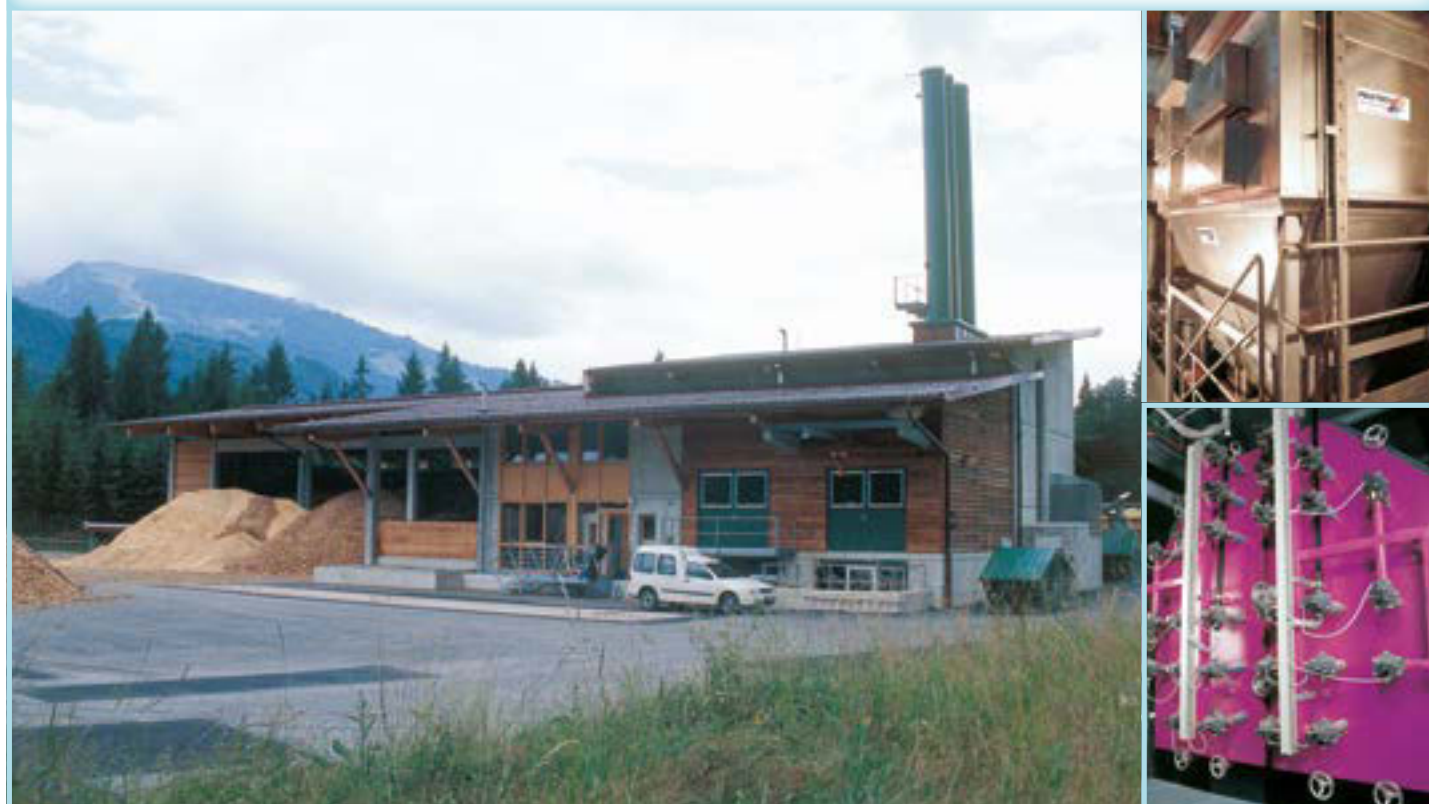
Combustion system: Water-cooled reciprocating grate • Fuel: Wood chips, forest residues and bark • Commissioned in 2000
