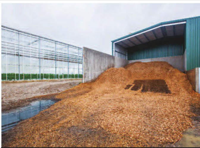
Fuel bunker with automatic walking floor.
